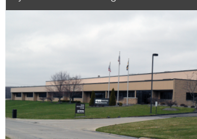
Wadsworth, OH - Industrial Profile Systems manufacturing.
