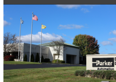
Irwin, PA - Mechanics Business Unit and manufacturing.
